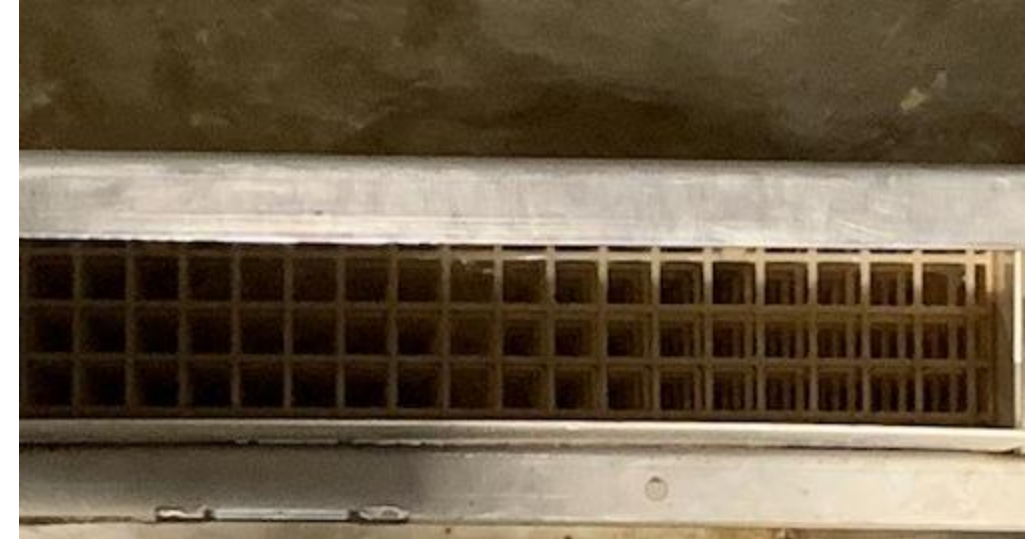
Degasser in use at Vikan Settefisk Zero biofouling In use ca 3 months
